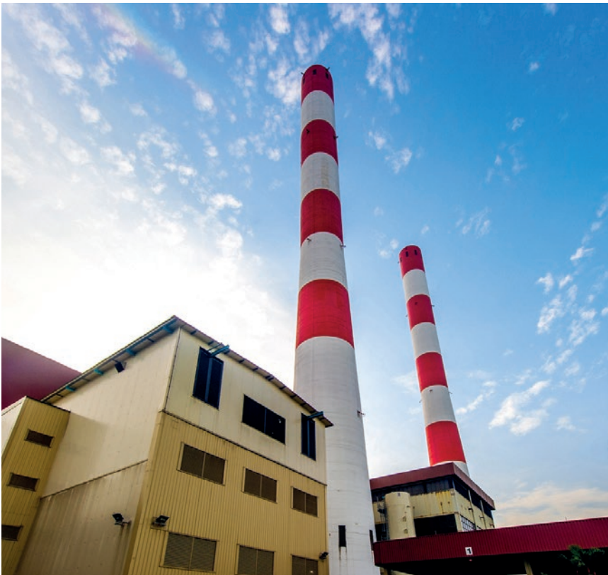
A significant amount of water is recycled at the Senoko WTE Plant (pictured) through an innovative process of treating effluent water from the refuse leachate and wastewater.
