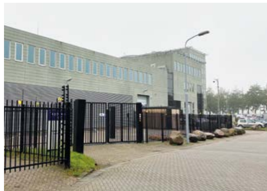
Amsterdam Data Centre is located in the Schiphol-Rijk business park where the Amsterdam Internet Exchange has a point of presence.
