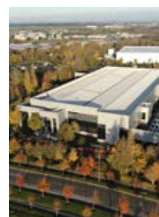
Keppel DC Dublin 1
