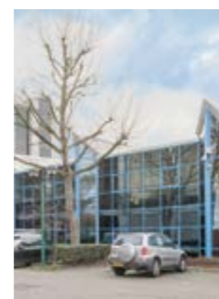
GV7 Data Centre
