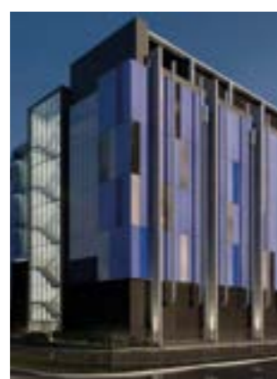
Intellicentre 3 East Data Centre (Under development)
