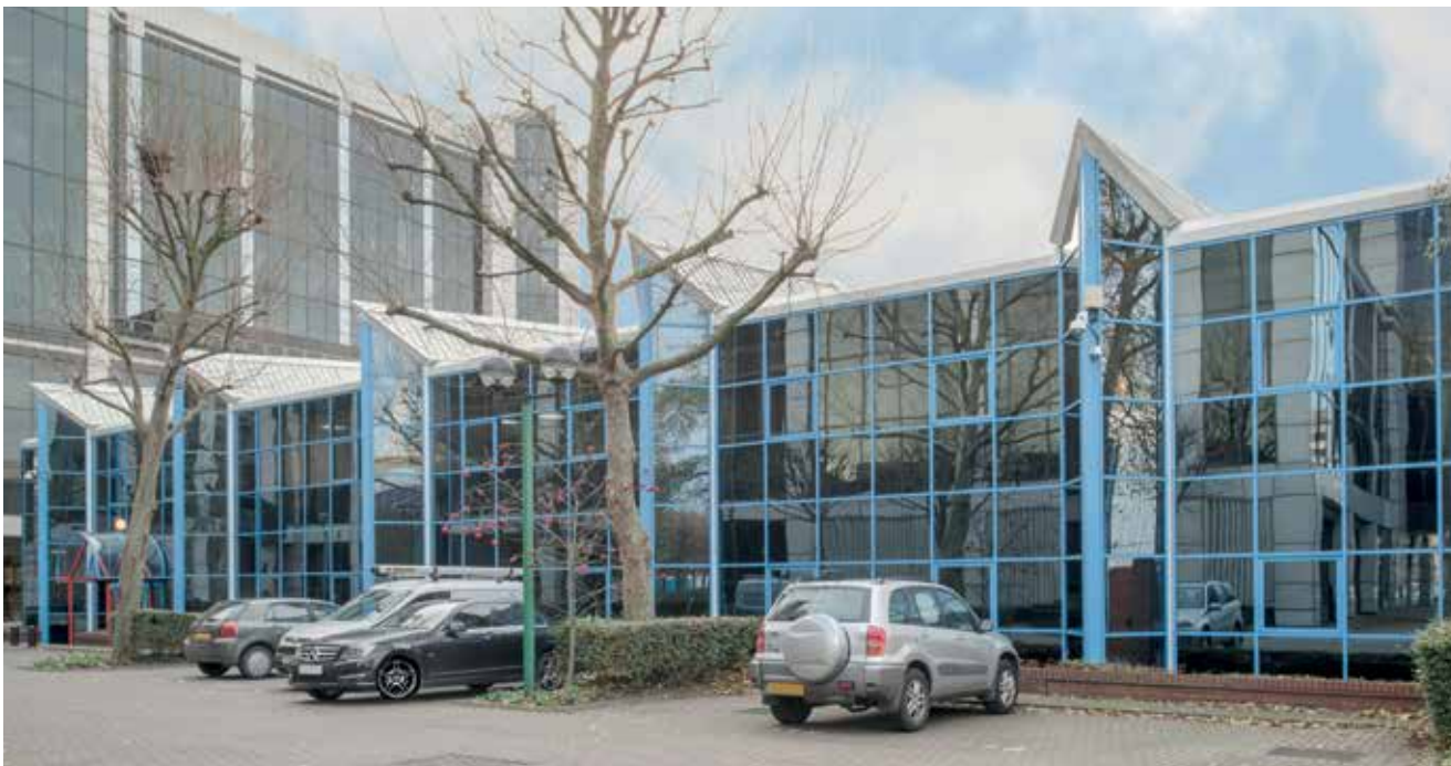
GV7 Data Centre is located in Greenwich View Place in London.
