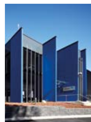
Intellicentre 2 Data Centre
