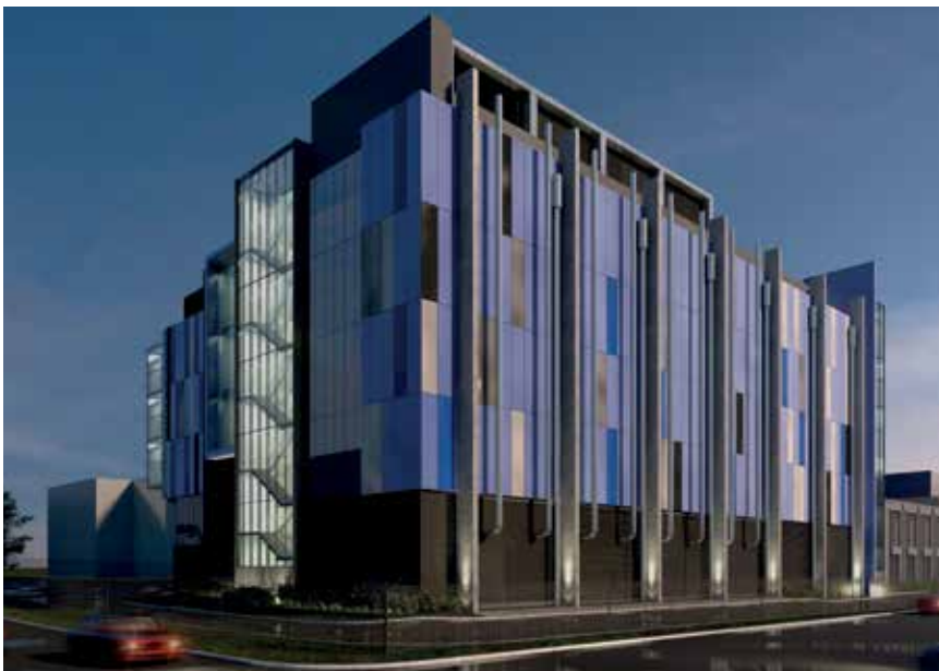
Intellicentre 3 East Data Centre in Sydney, Australia, is on track for completion in 1H 2021.
