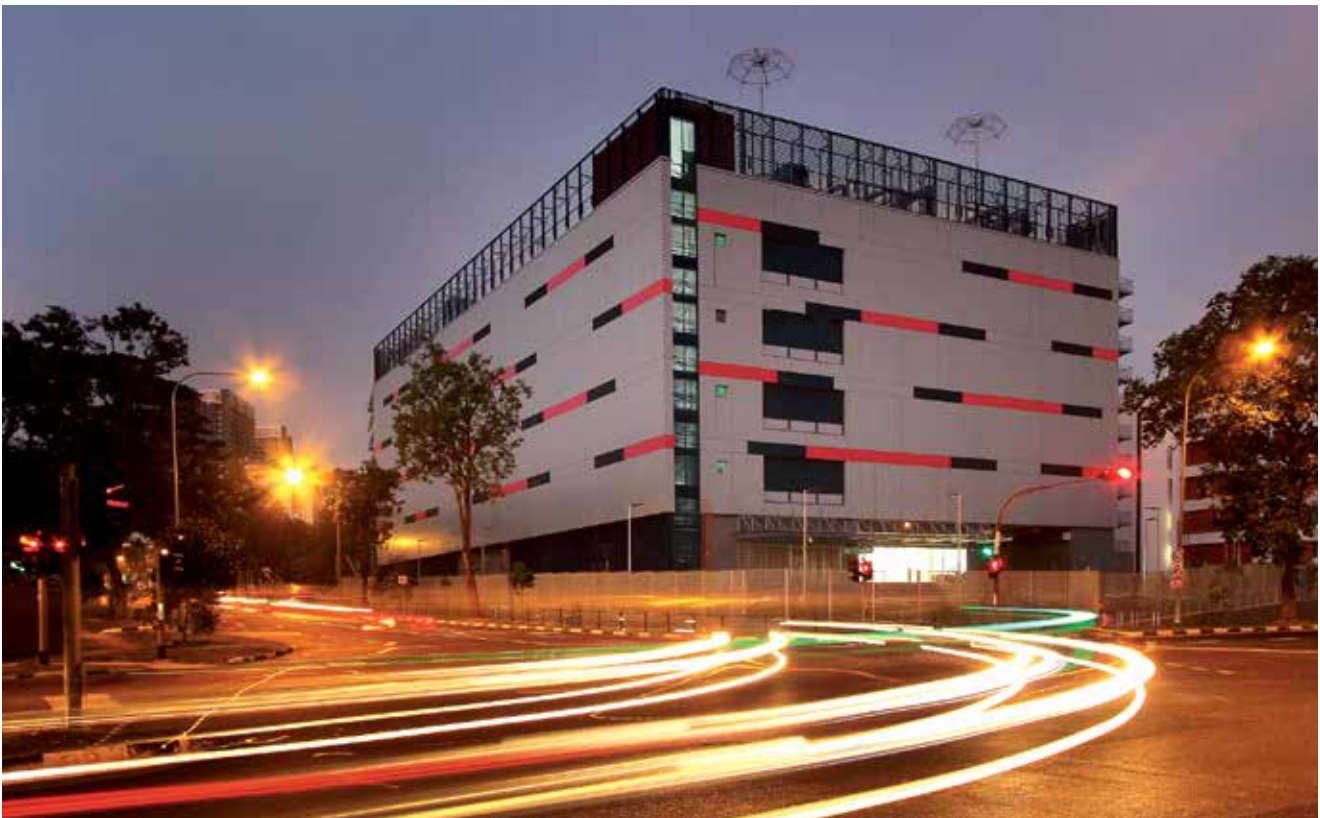
Distribution income for FY 2020 included full year contributions from Keppel DC Singapore 4 and DC1 (pictured), as well as the REIT's new acquisition of Kelsterbach Data Centre.
