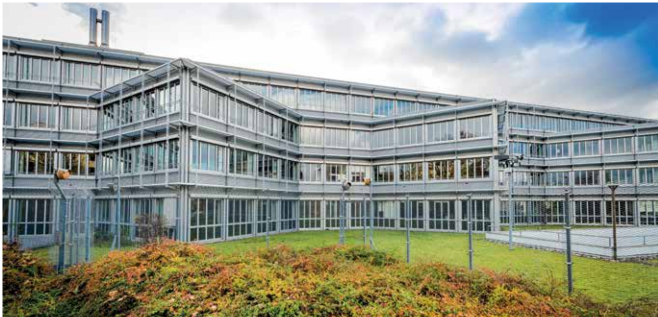
Kelsterbach Data Centre is located near the Frankfurt airport and approximately 18km from the Frankfurt city centre.
