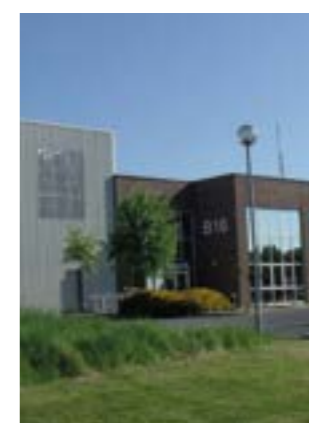
Keppel DC Dublin 2
