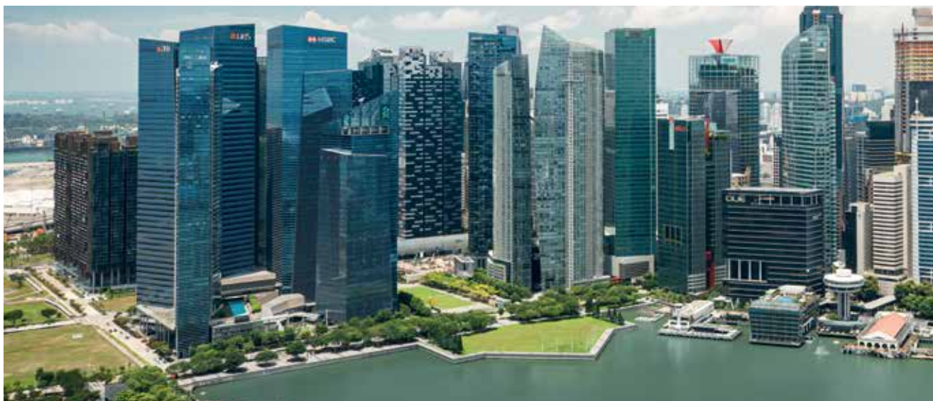
Singapore is a choice location for multinational organisations due to its robust fibre network, pro-business climate and competitive power market.
