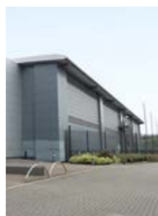
Cardiff Data Centre
