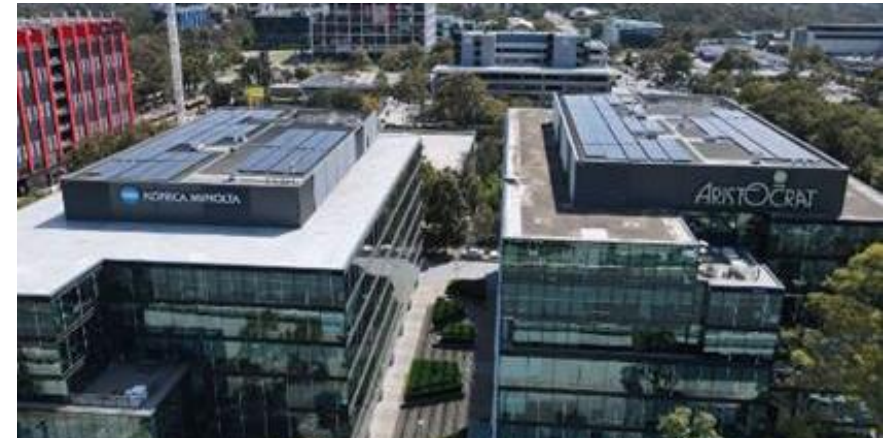
Solar panels were installed at Pinnacle Office Park in Dec 2021 to tap on renewable energy
