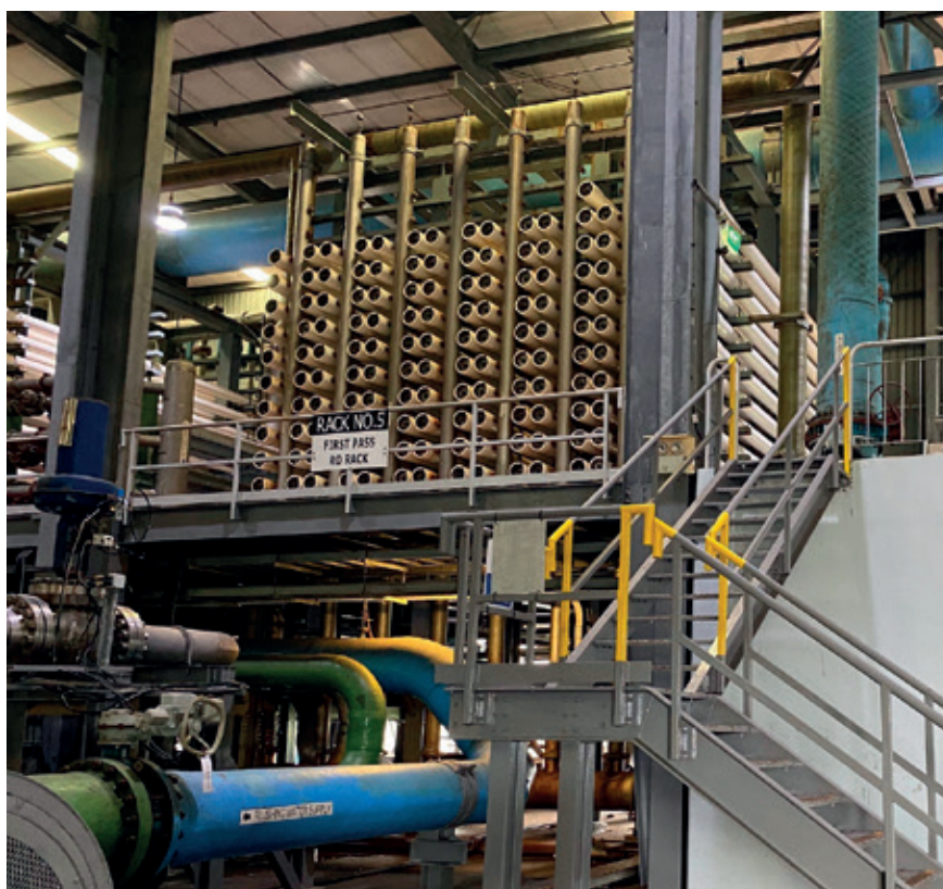
The SingSpring Desalination Plant was the largest membrane-based seawater desalination plant in the world at the time of its completion.
