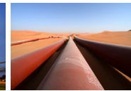
Aramco Gas Pipelines Company (AGPC)
