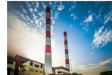
Senoko Waste-to-Energy (WTE) Plant
