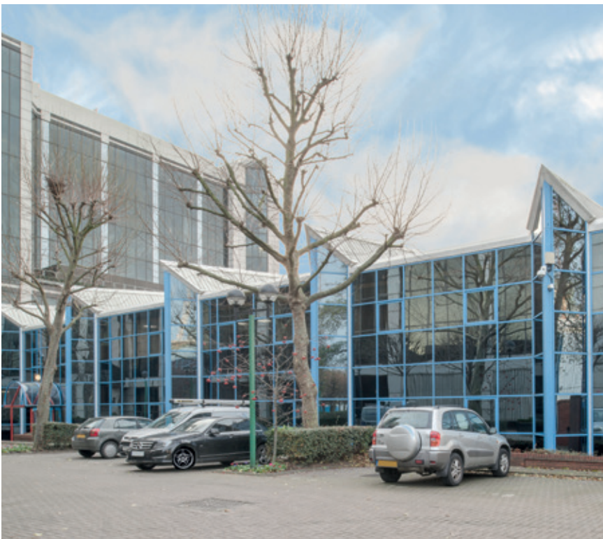
GV7 DC is located in Greenwich View Place, a data centre hub with many operators offering high connectivity services.
