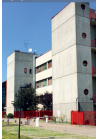
Milan Data Centre
