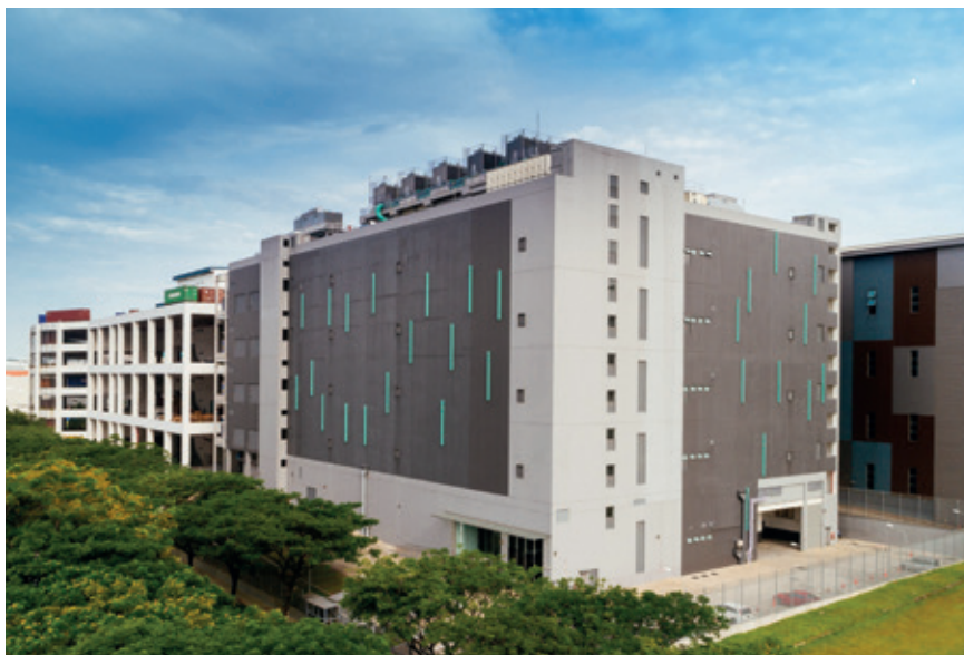
Keppel DC Singapore 5 is located in Jurong, one of the largest clusters of data centres in Singapore.
