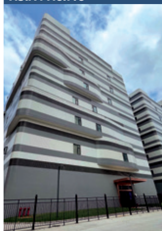
Guangdong Data Centre 1
