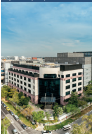
Keppel DC Singapore 1
