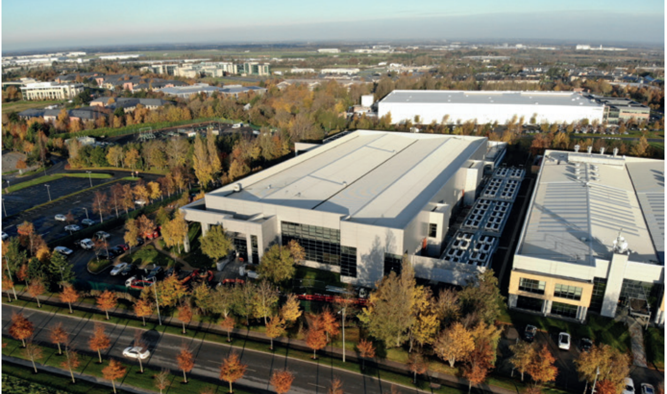
Keppel DC Dublin 2 is an energy-efficient colocation data centre located in the Citywest Business Campus, a prime suburban industrial and commercial location.
