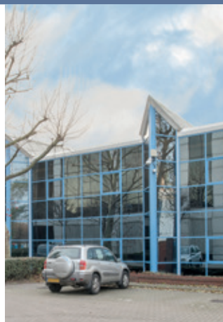
GV7 Data Centre
