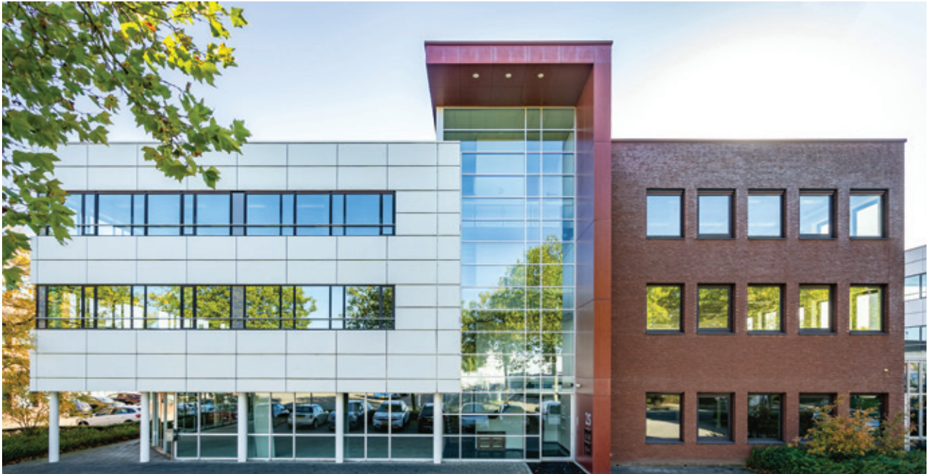
Eindhoven DC comprises two shell and core data centre buildings as well as a warehouse and an ancillary office building in De Hurk, the largest business park in Eindhoven, the Netherlands.
