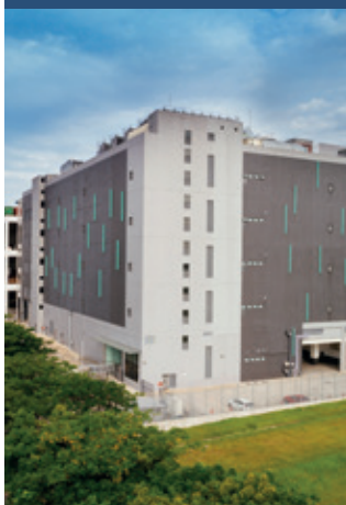
Keppel DC Singapore 5
