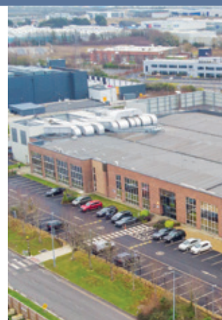
Keppel DC Dublin 2
