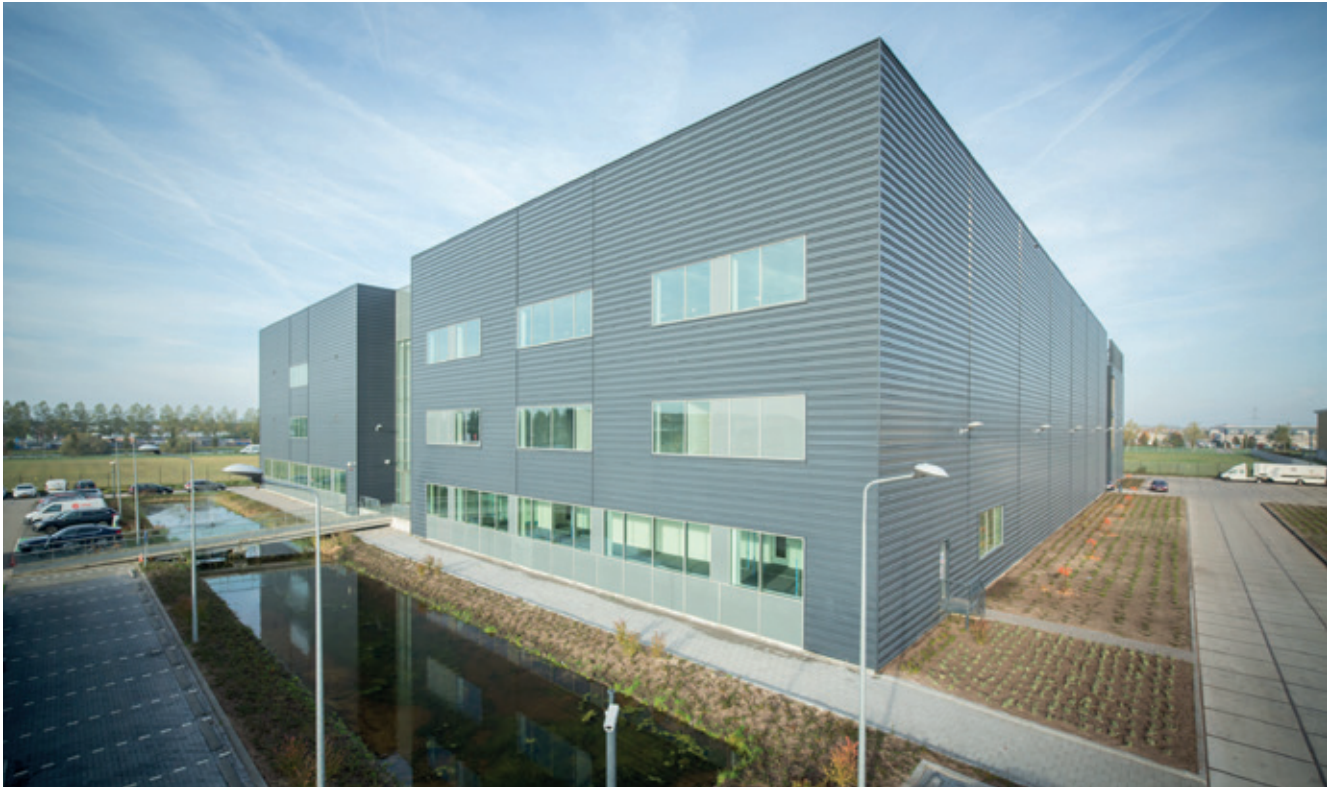
Almere DC is located in the Sallandsekant business park, in the city of Almere, the Netherlands.
