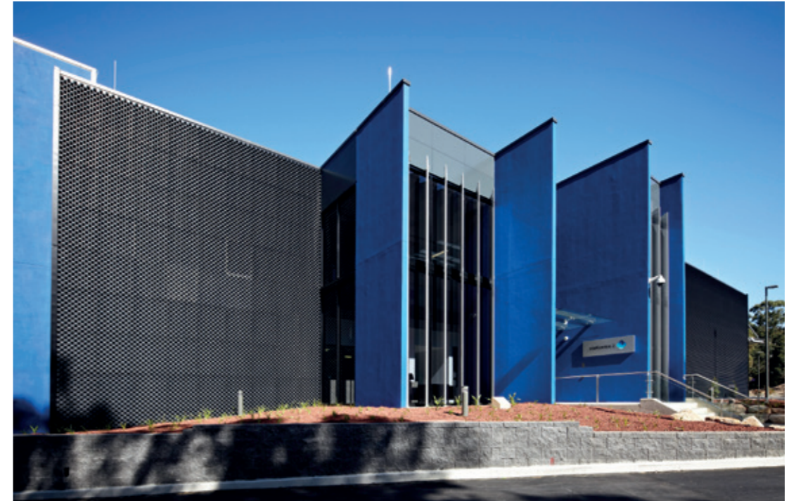
The Manager will actively manage and optimise the portfolio, leveraging Keppel’s unique proposition of operational and technical expertise to create value in a constantly changing world.
