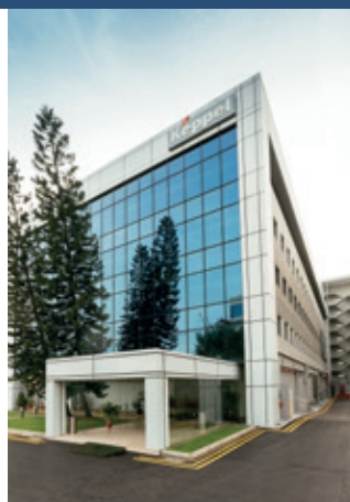
Keppel DC Singapore 2
