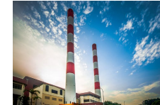
Senoko Waste-to-Energy (WTE) Plant
