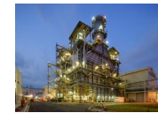
Keppel Merlimau Cogen Plant (KMC)
